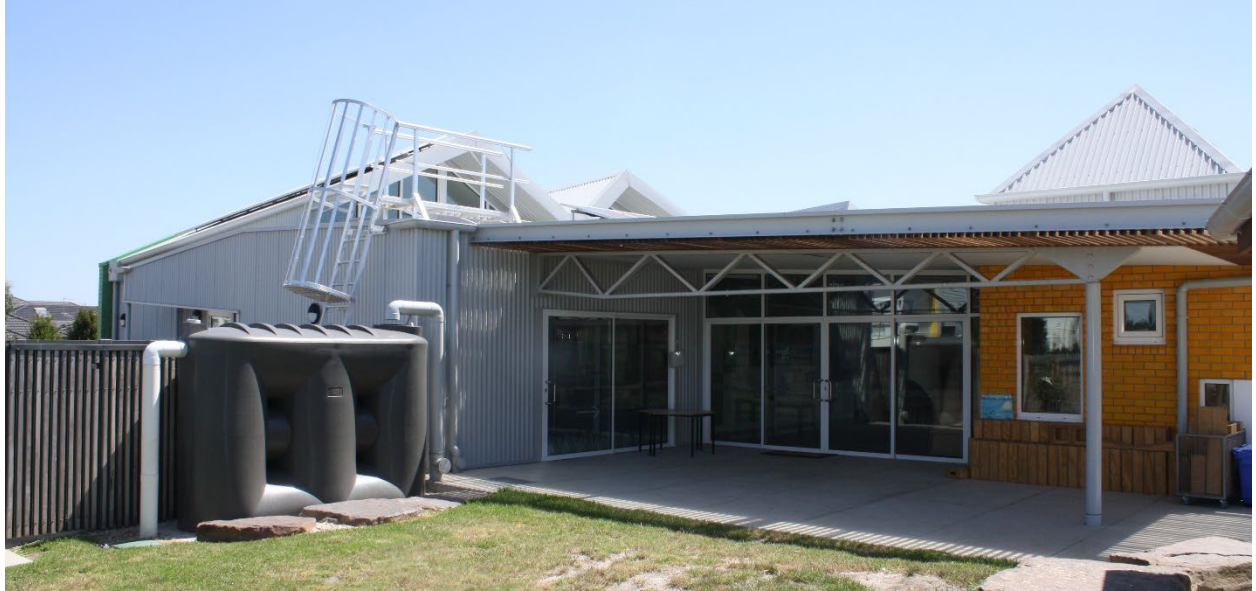
Image 4: Arena Family and Child Centre rainwater tank
