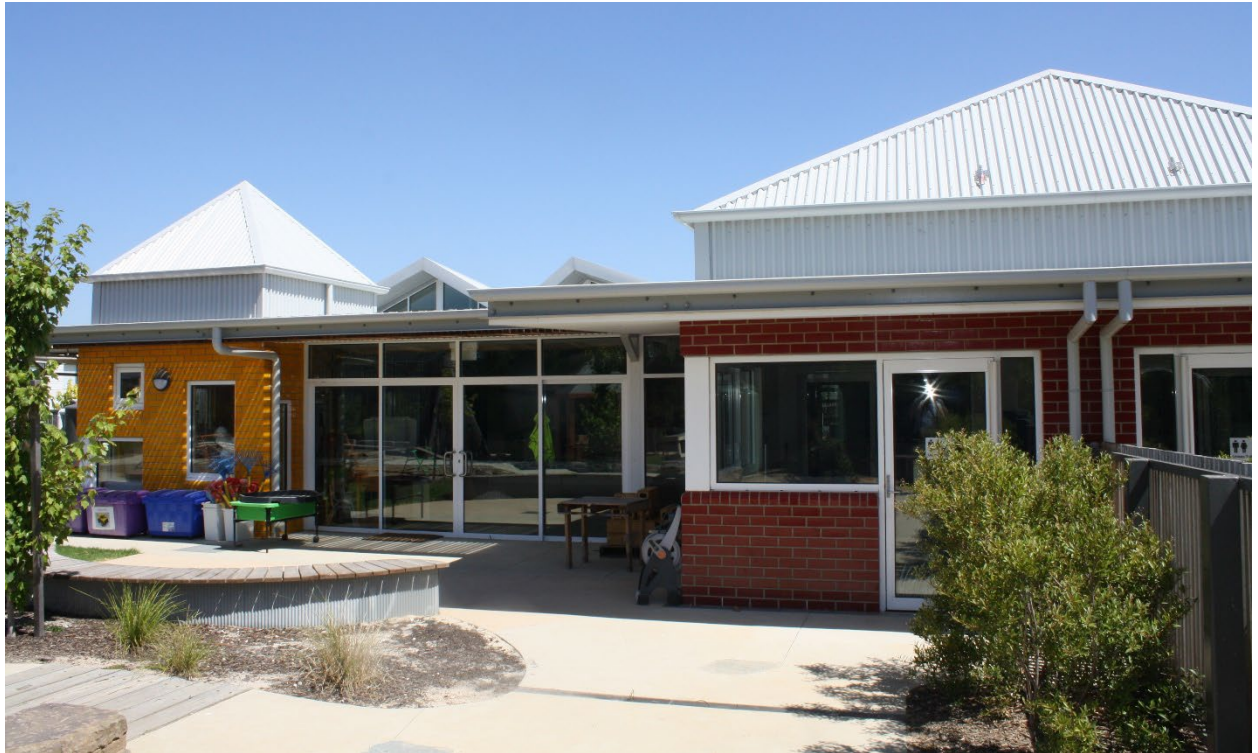
Image 3: Arena Children's Centre Northern facade
